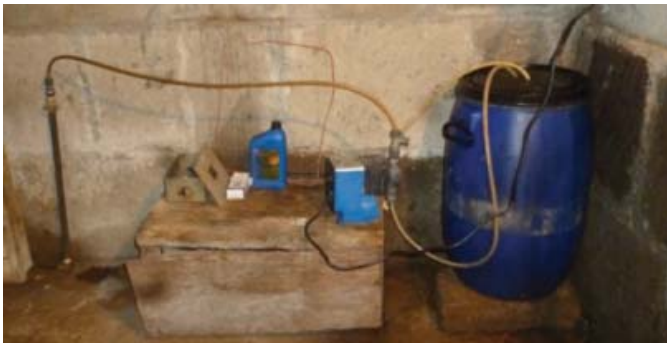
Previous chlorinator method in México.
